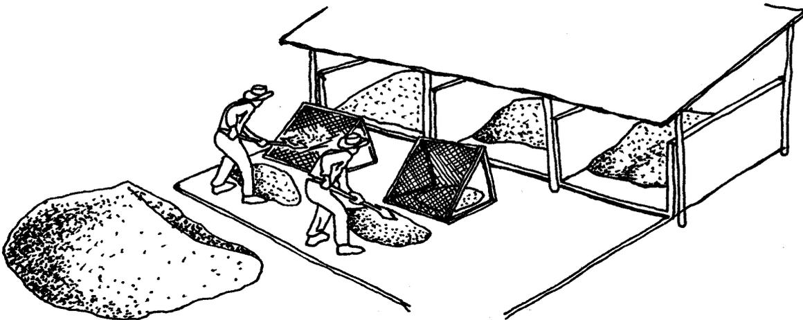
Sand should be **stored under cover** so that rain and damp do not add too much water to the sand.
